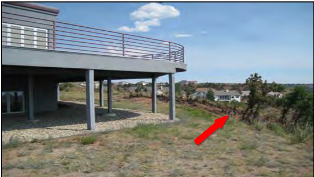
Figure 37 – Example of how understory vegetation burned but did not burn the canopy of the trees and due to mitigation efforts, did not burn the structure.
