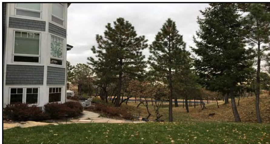
Figure 28 – Example of properly mitigated vegetation within the safety zone
