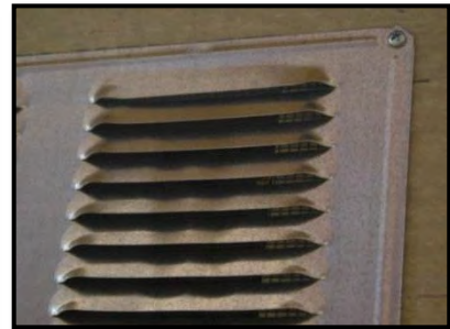
Figure 13 – Example of a roof vent.
