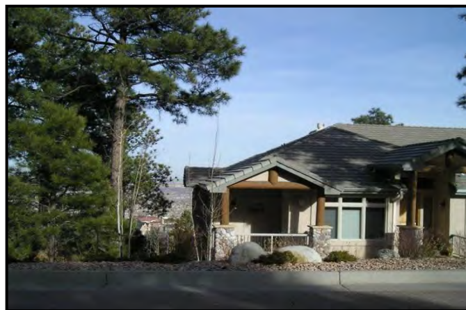
Figure 40 – Example of a home that has pruned branches from the roofline of their home.
