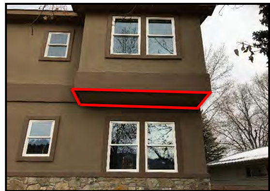
Figure 8 – The red lines depict the areas that would be required to be built of ignition resistant materials
