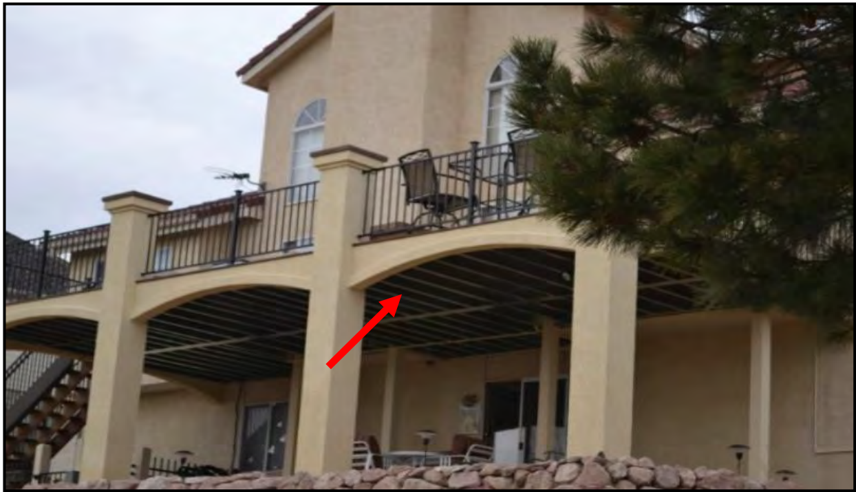
Figure 22 – The arrow depicts the metal floor joists used on this example deck.
