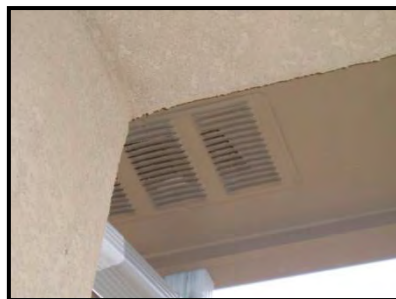
Figure 12 – Example of a soffit vent.
