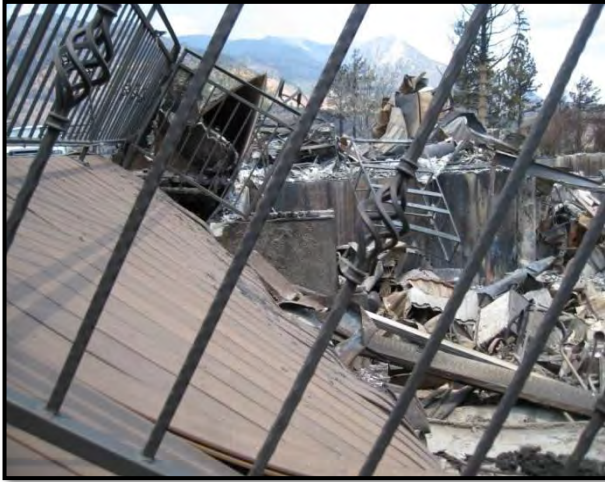
Figure 20 – Example of composite decking after the structure was lost during the Waldo Canyon Fire
