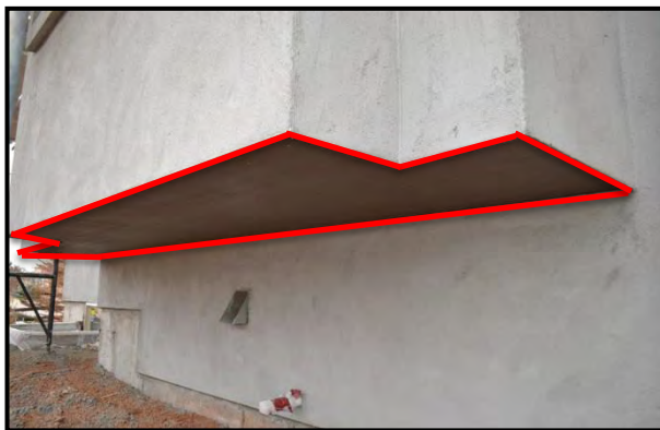
Figure 8 – The red lines depict the areas that would be required to be built of ignition resistant materials
